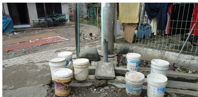
PNPM SUPPORTED WATER AND DRAINAGE IMPROVEMENTS TO SLUM AREAS
